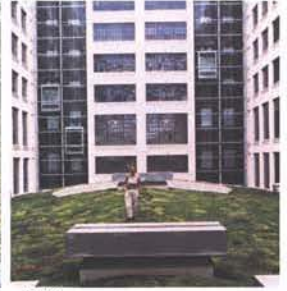
SEDUM GREEN ROOF - EAST COURTYARD
